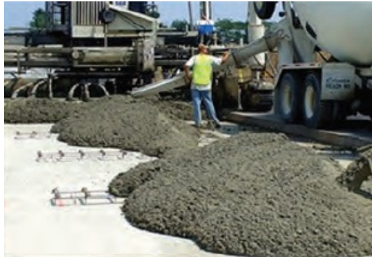
Lightweight Ready-mix, Concrete & Industrialized Building System (IBS)
